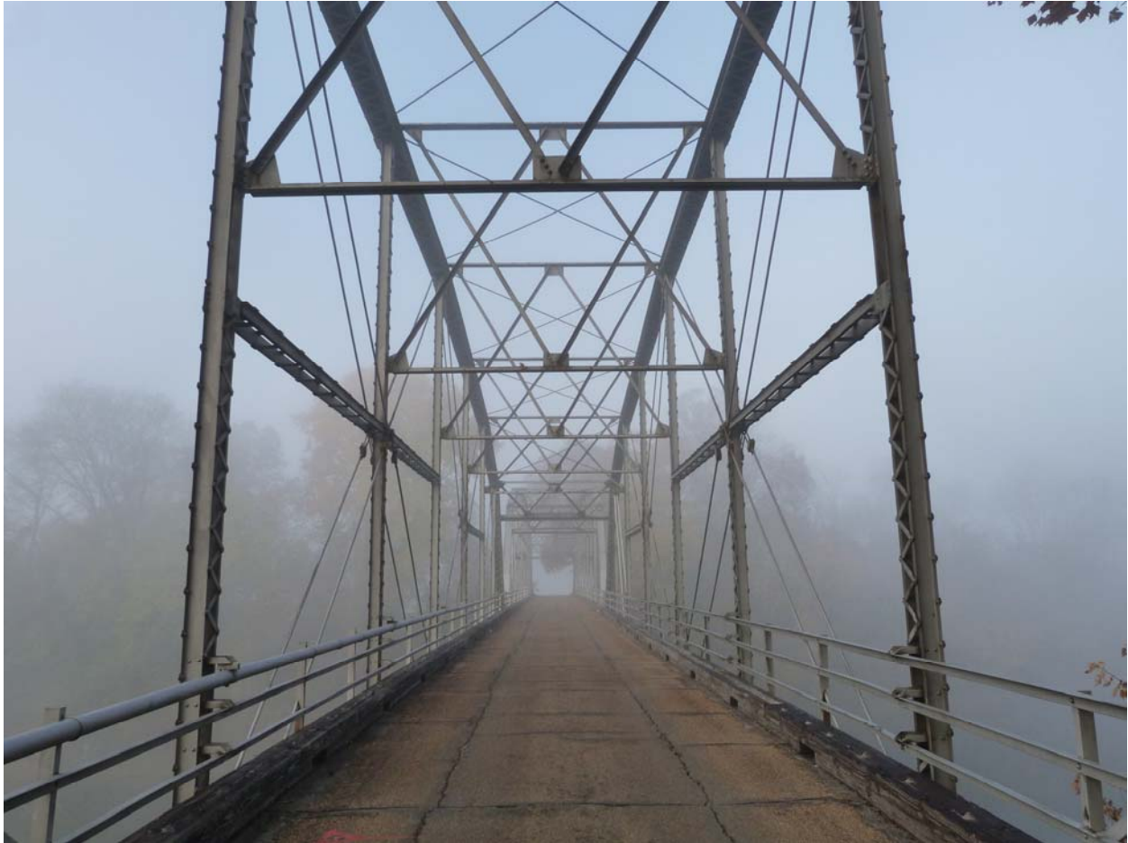
8 – Standing on the bridge deck.
