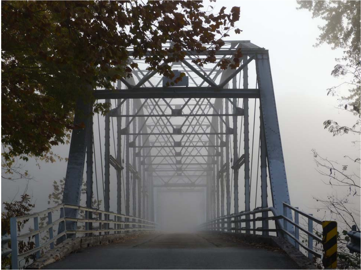
2- Portal view of the bridge.
