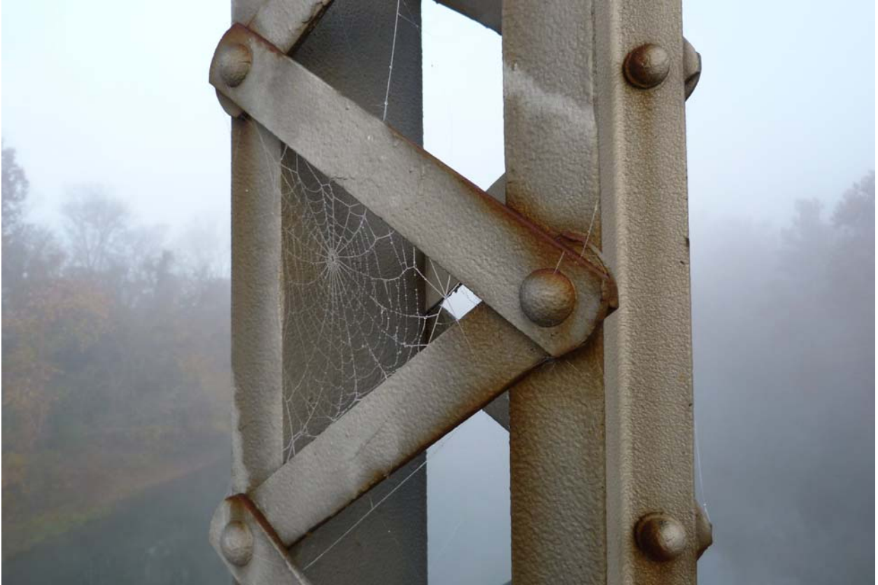
7- A spider web on a vertical member of the bridge.
