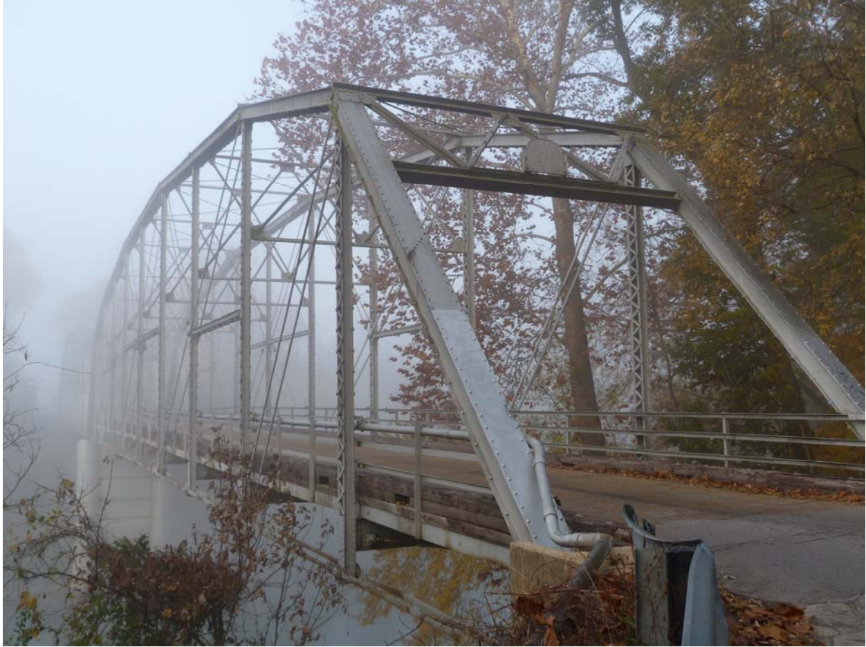
1 – Oblique view of the bridge.
