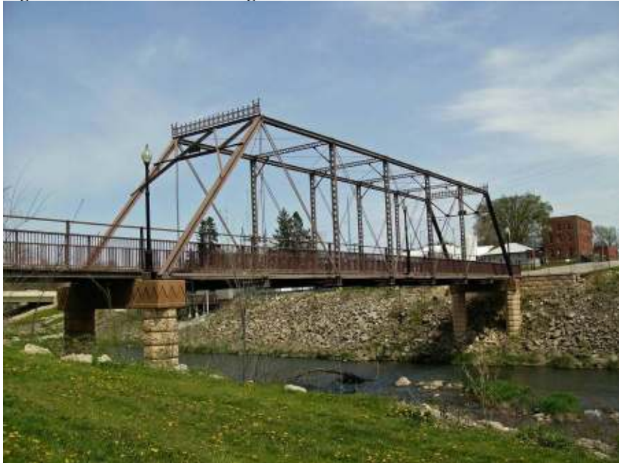
Figure 15. Walnut Street Bridge
