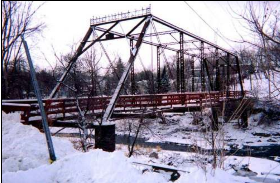
Figure 14. Walnut Street Bridge
