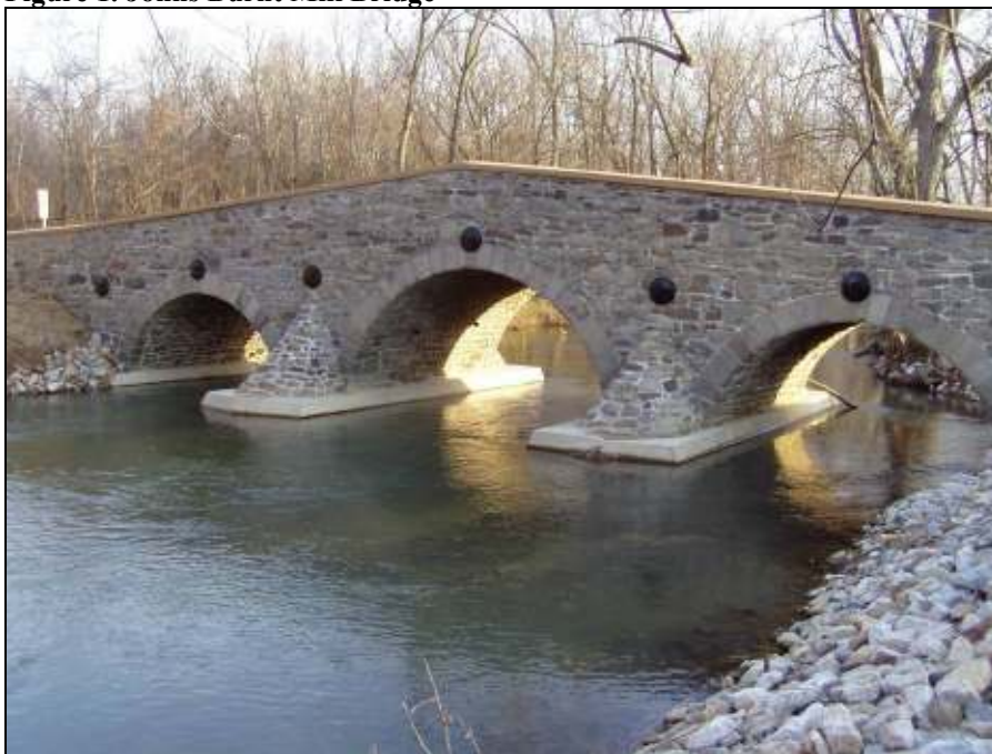
Figure 1. Johns Burnt Mill Bridge
