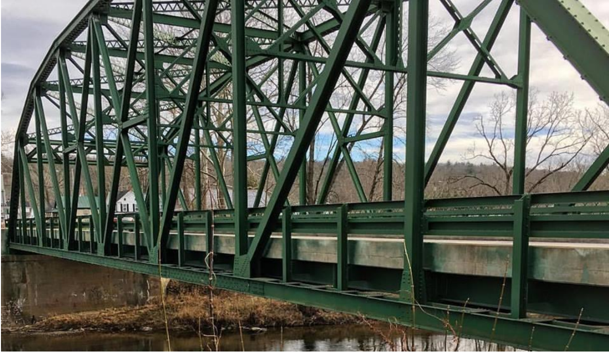
Overview of the bridge.
