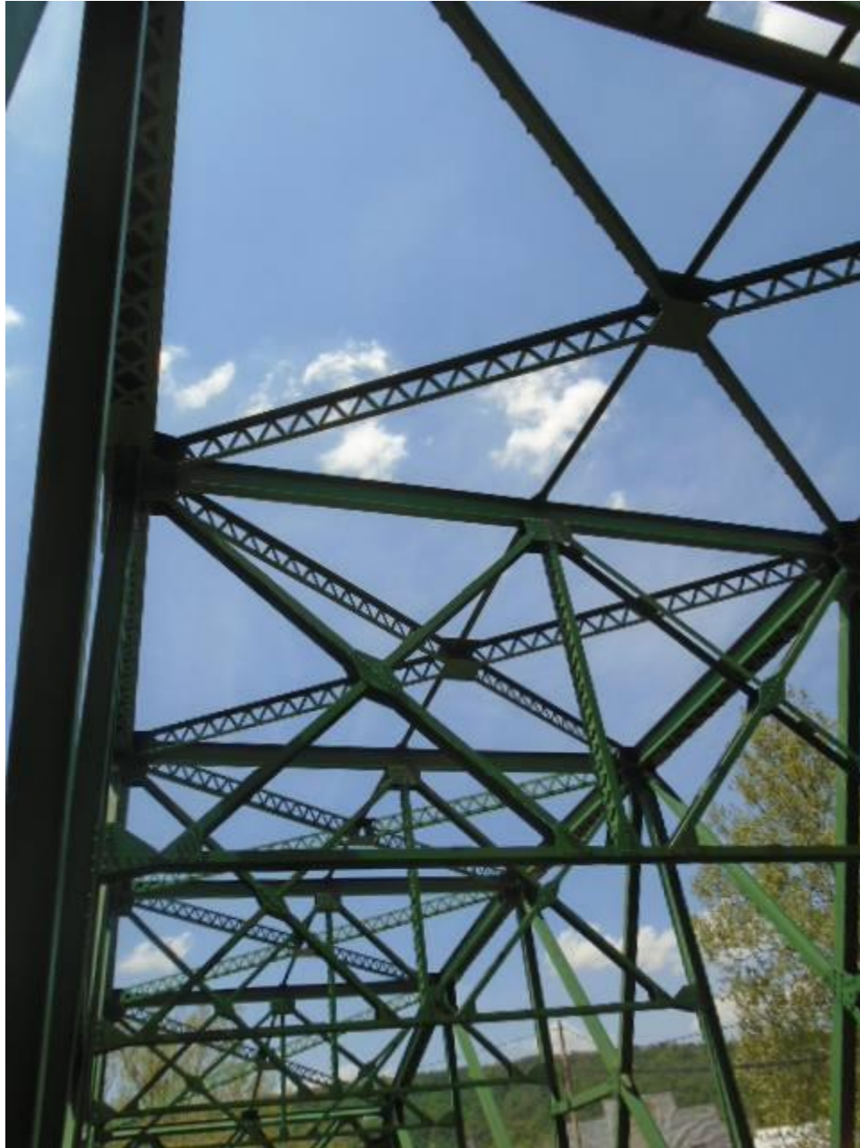
Overhead sway bracing and lateral bracing on bridge.
