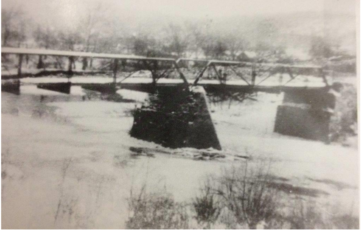
One of the earlier bridges at this location, a metal Pratt pony truss bridge with pinned connections.
