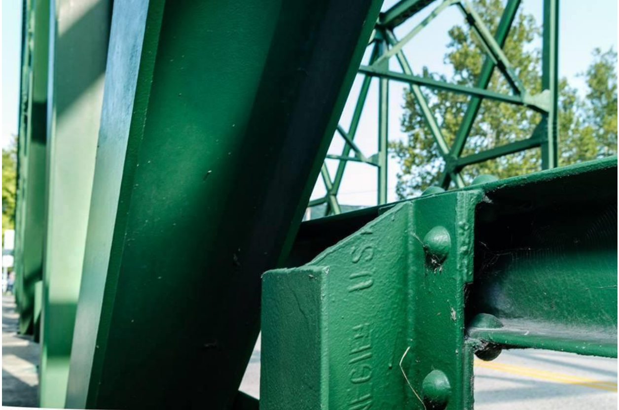
Detail with a Carnegie brand visible on the railing support.
