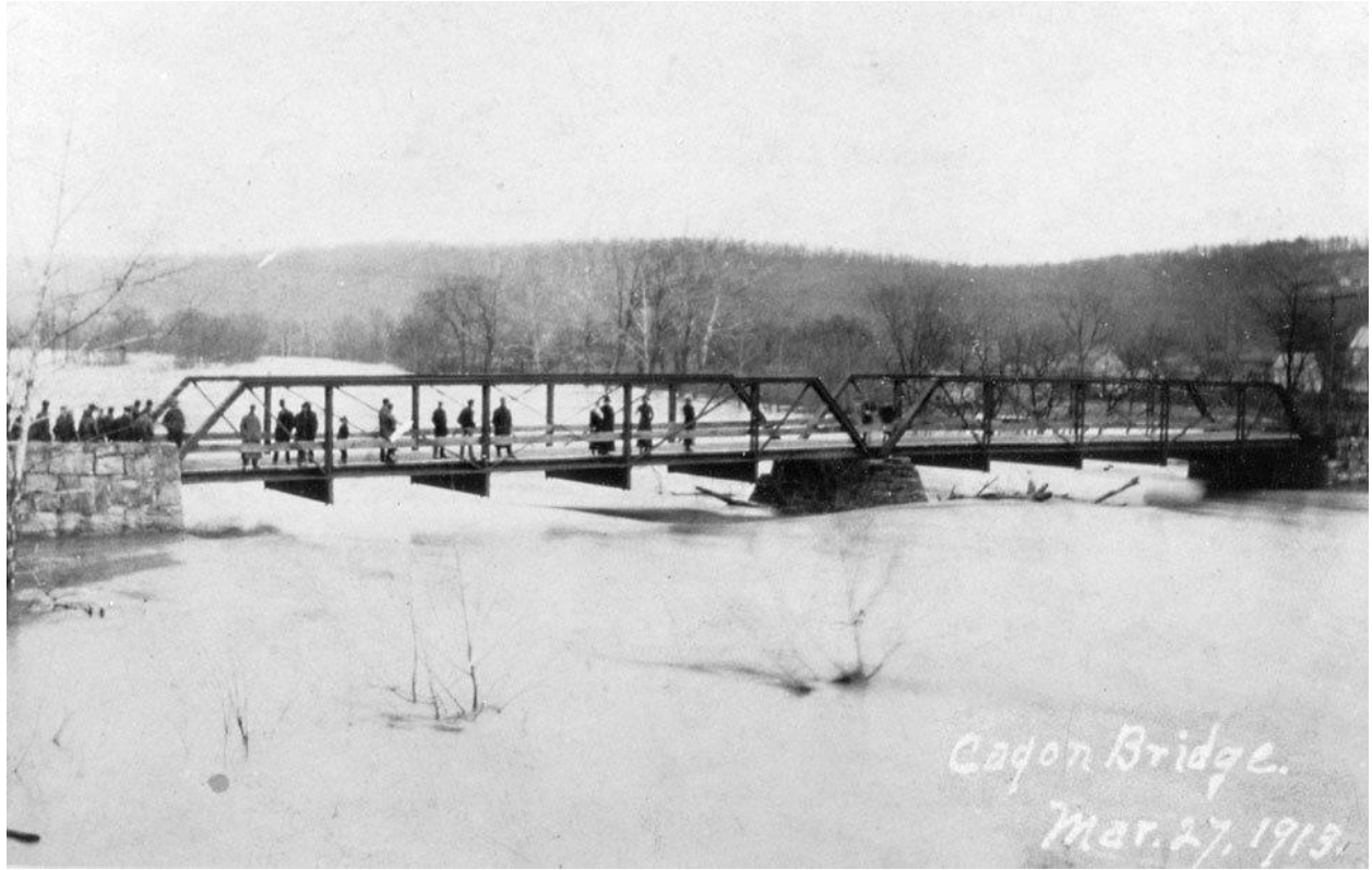
One of the earlier bridges at this location, a metal Pratt pony truss bridge with pinned connections.
