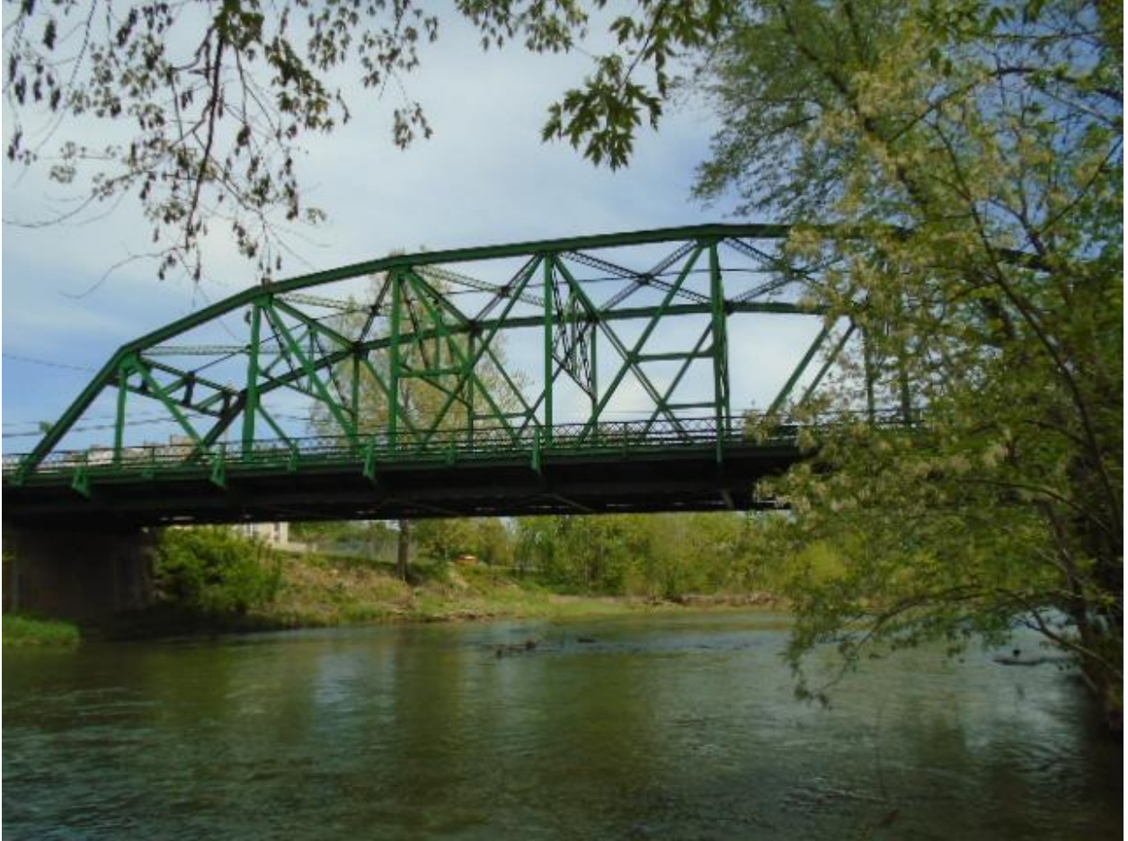
Overview of the bridge.
