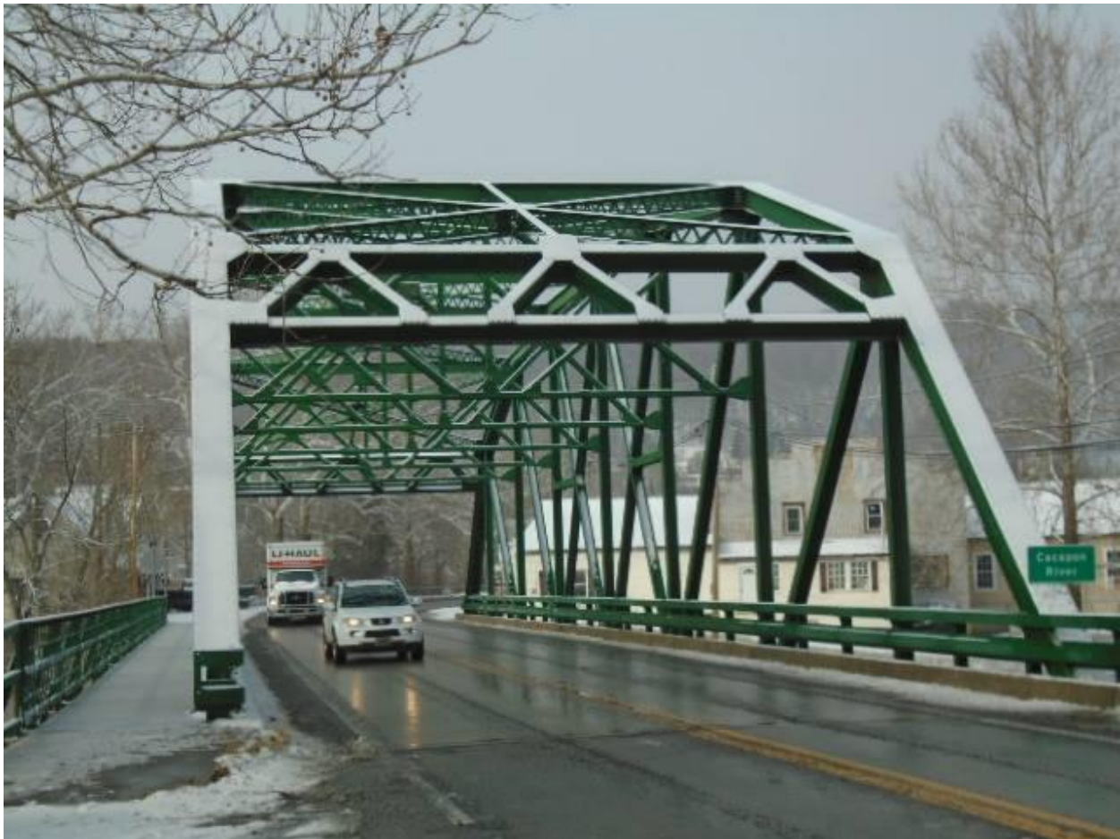
Overview of the bridge.
