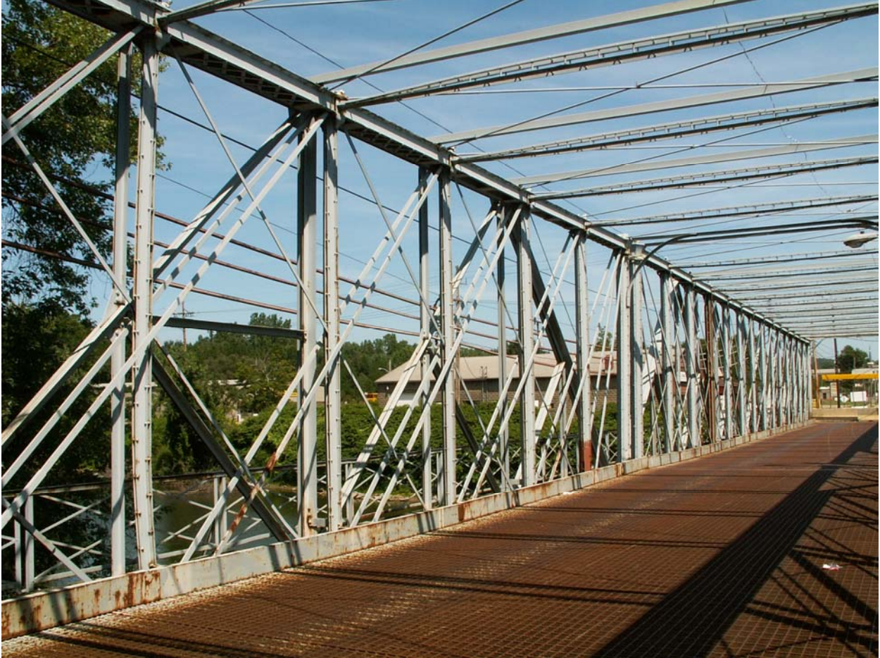
View of the truss webs.
