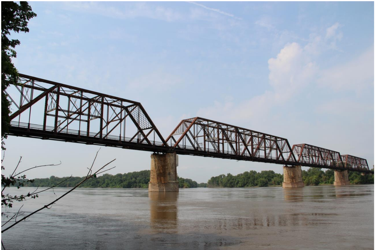
Top: Merchants Bridge. Bottom: Bellefontaine Bridge
