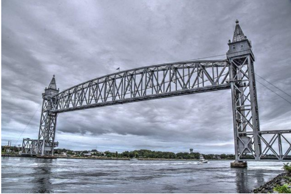
Cape Cod Canal Railroad Bridge in Buzzards Bay, Massachusetts
