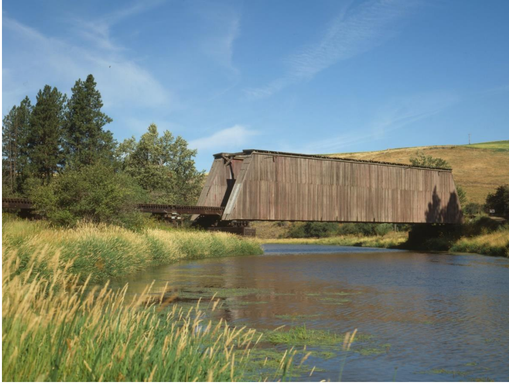
Goodpasture Covered Bridge
