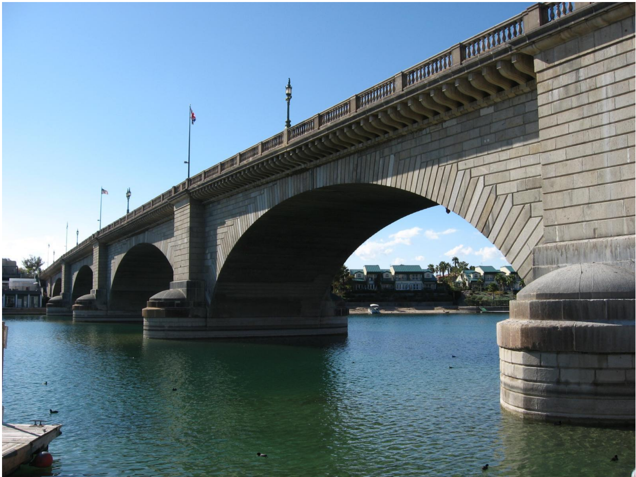
A photo of London Bridge at Lake Havasu.
