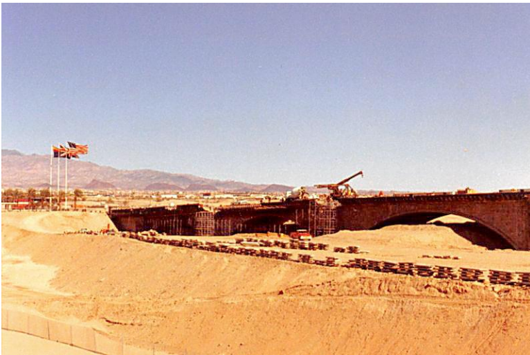
Construction of London's Bridge at Lake Havasu in 1971.
