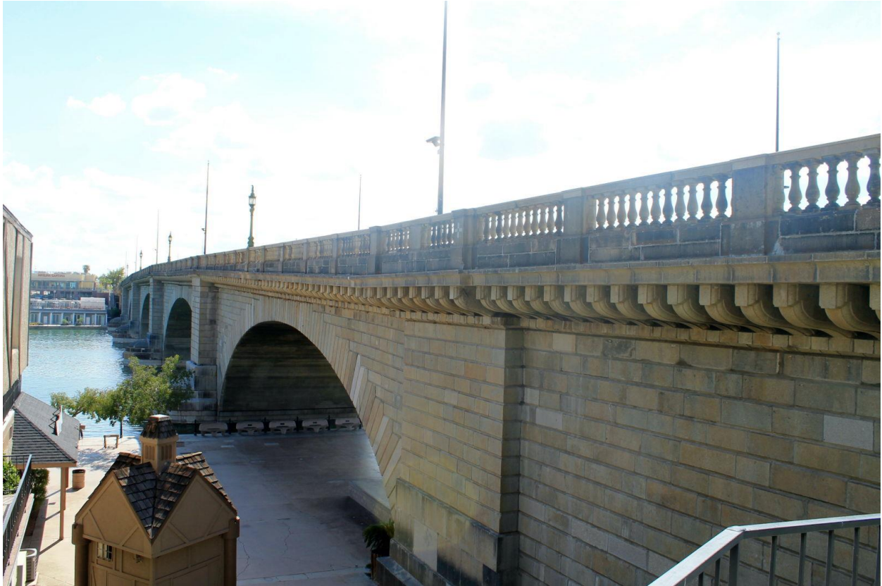
A photo of London Bridge at Lake Havasu.
