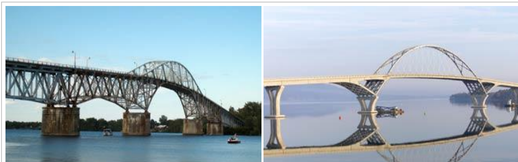
One large span, rising high above the lake's navigational channel, is a strikingly similar feature of the 1929 and 2011 Lake Champlain Bridge. Image (right) © Andy Ryan, photo courtesy of HNTB
