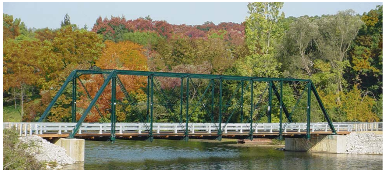
The Maple (Foster) Road Bridge as it exists today.
